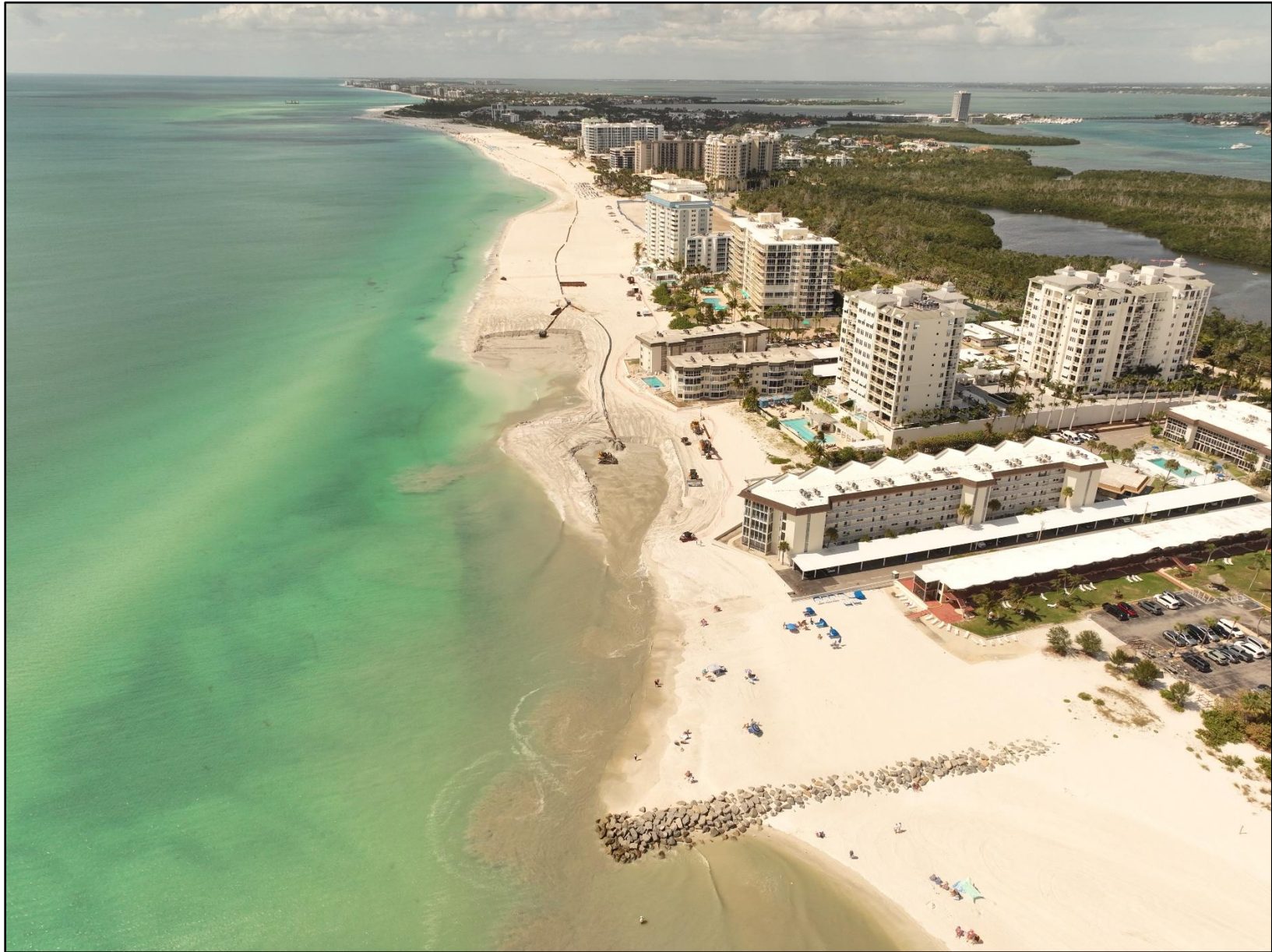
Project Photo 6. Lido Key Shore Protection Project being constructed in April 2026, near R42 and R43. Photo courtesy of Morjana Signorin, P.M., with Coastal Protection Engineering (CPE). See additional construction photos of beach nourishment projects.
