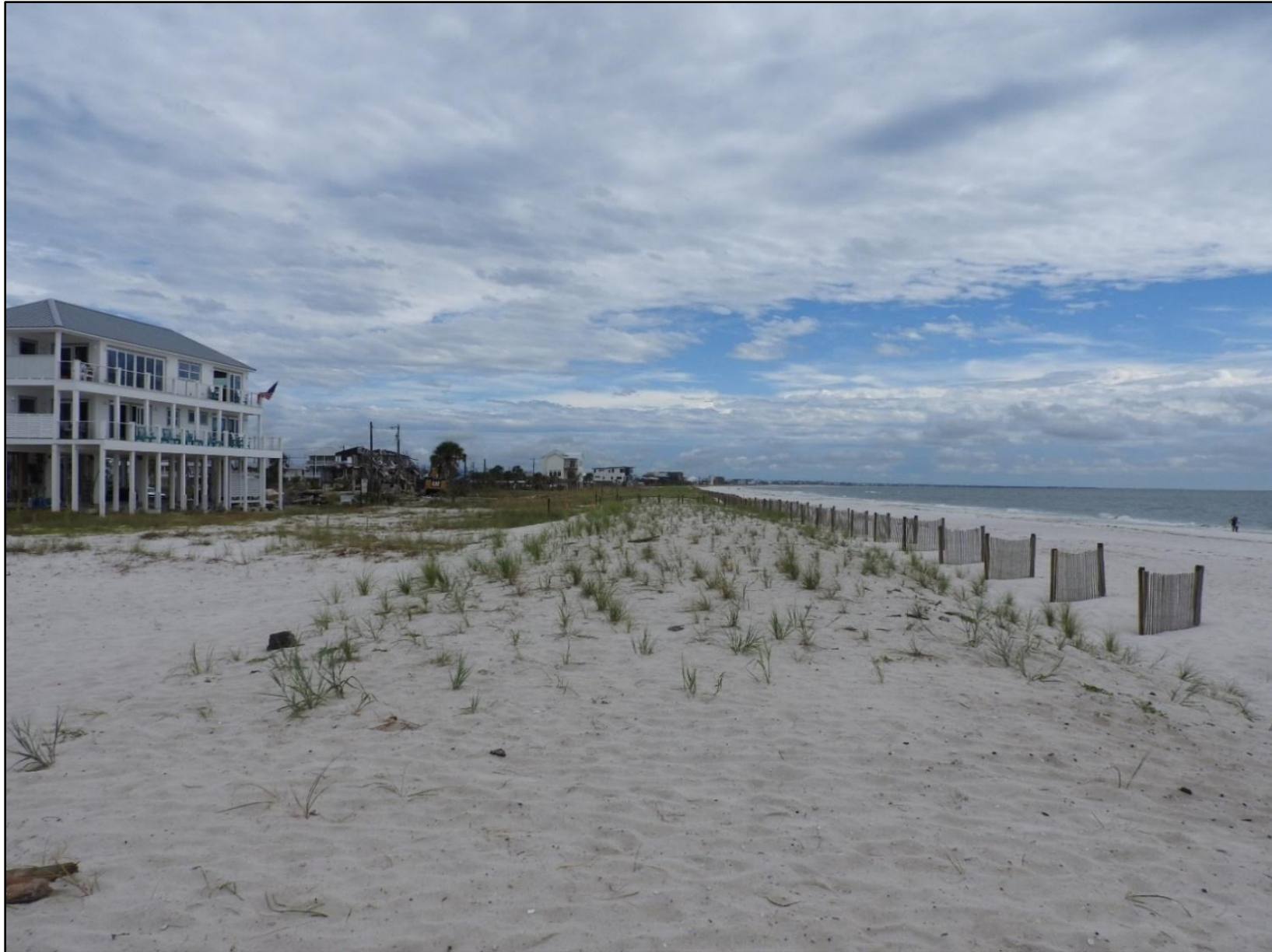
Figure 9. Mexico Beach, with a newly constructed FEMA dune/berm in 2019, post-Hurricane Michael (2018). The FEMA dune/berm is located between the inlet (R128) and the Bay/Gulf County line (R144). DEP file photo taken in October 2019 by Guy Weeks.
