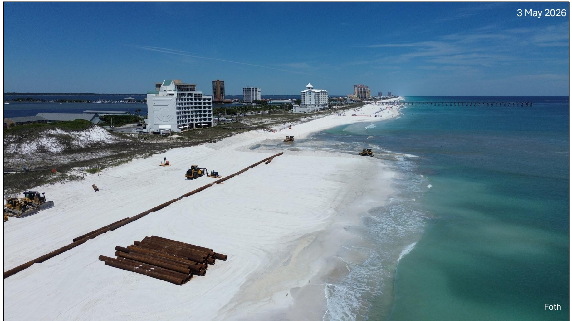
Project Photo 1. The Pensacola Beach Nourishment Project being constructed in May 2026 and sponsored by the Santa Rosa Island Authority.
