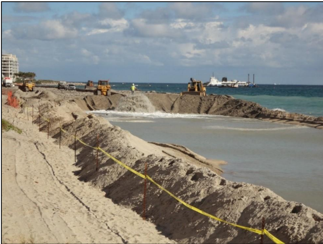
Figure 15. South Boca Raton beach nourishment project (2013) using sand from offshore sources. Photo courtesy of Peter Seidle, P.E.
