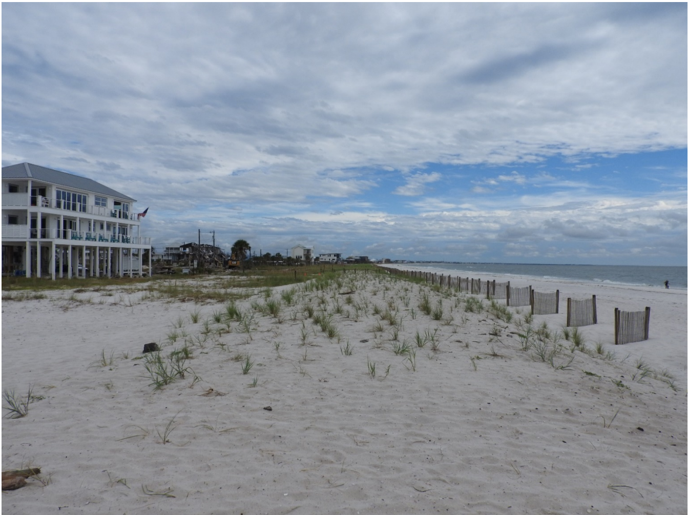
Figure 2. Mexico Beach with a newly constructed FEMA dune/berm in 2019, post-Hurricane Michael (2018). The FEMA dune/ berm is located between the inlet (R128) and the Bay/ Gulf County line (R144). Department file photo taken in October 2019 by W.G. Weeks.
