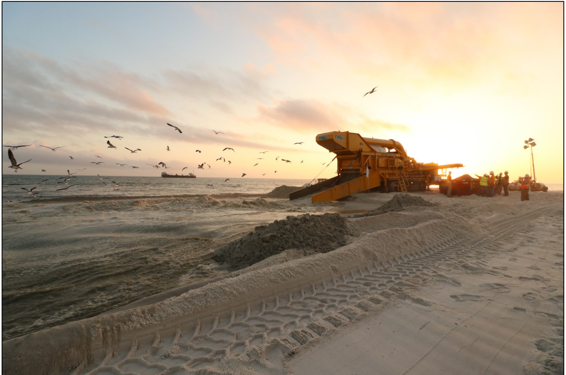
Panama City Beach Shore Protection Project under construction in March 2017. Photo courtesy of Bay County, Lisa Armbruster.
