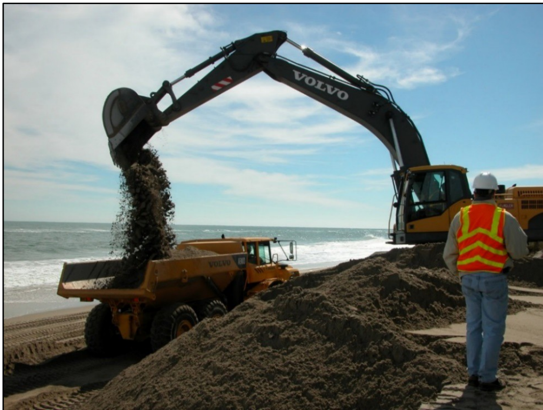
Figure 12. Wabasso Beach (Indian River County) nourishment project (Sector 3) using sand from upland sources. DEP project file photo (2010).
