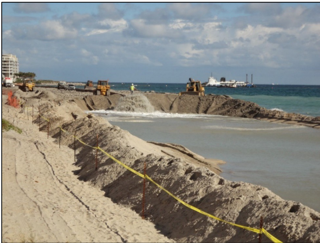
Figure 13. South Boca Raton beach nourishment project (2013) using sand from offshore sources. Photo courtesy of Peter Seidle, P.E.
