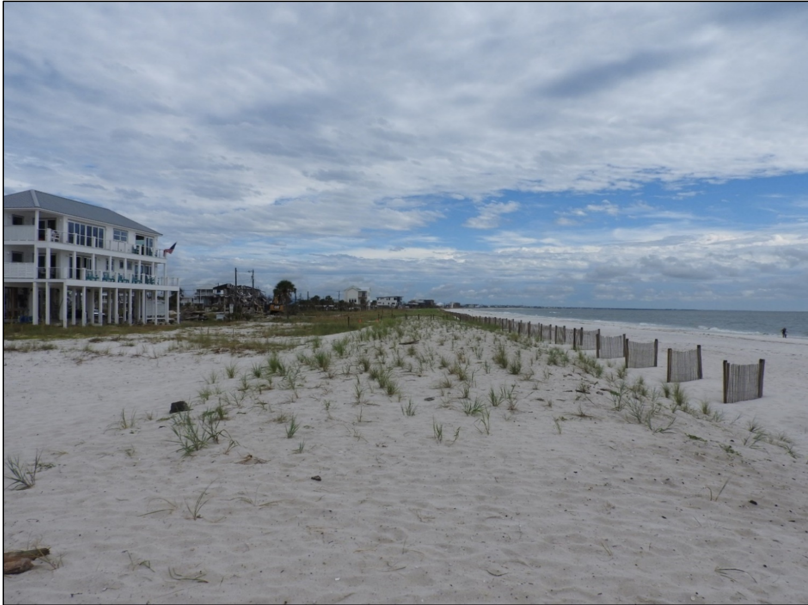
Figure 8. Mexico Beach, with a newly constructed FEMA dune/berm in 2019, post-Hurricane Michael (2018). The FEMA dune/berm is located between the inlet (R128) and the Bay/Gulf County line (R144). DEP file photo taken in October 2019 by W.G. Weeks.
