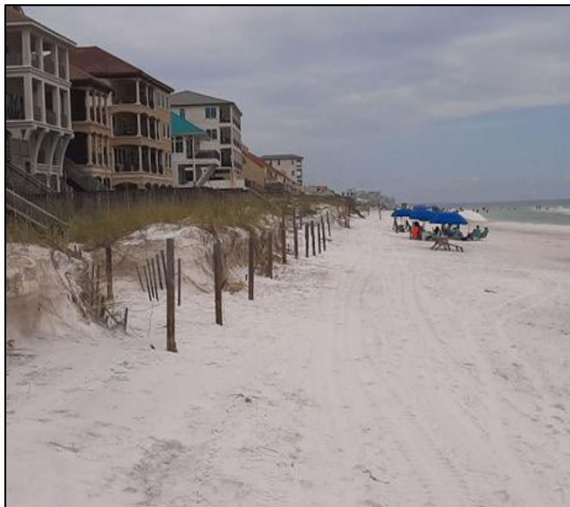
Figure 4. Condition II or Minor Dune and Beach Erosion is generally characterized by minor sandy beach deflation, or profile lowering, along with a 1-foot to 3-foot recession and vertical escarpment of the existing dune.
