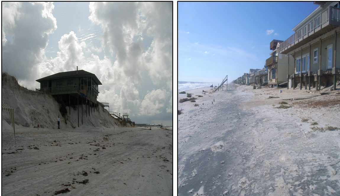
Figure 6. Condition IV or Major Dune Erosion is generally characterized by recession of the existing dune along with a vertical escarpment, or “cliffing,” in excess of 10 feet and a less-defined amount of beach deflation or profile lowering across the sandy beach. Condition IV may also include a complete loss or removal of a previously existing dune feature.
