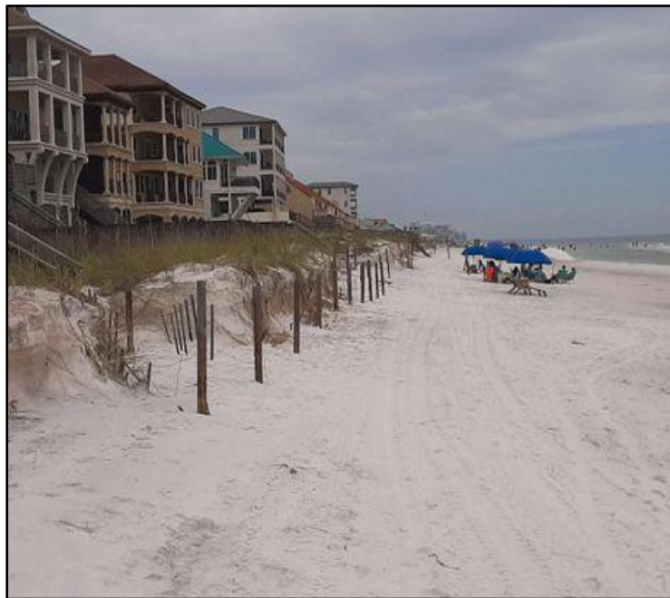
Figure 5. Condition II or Minor Dune and Beach Erosion.
