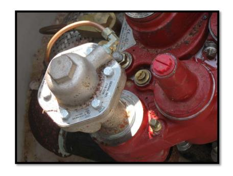
All new pressurized small diameter piping in contact with the soil must be installed with line leak detectors, and must be tested every 12 months.
