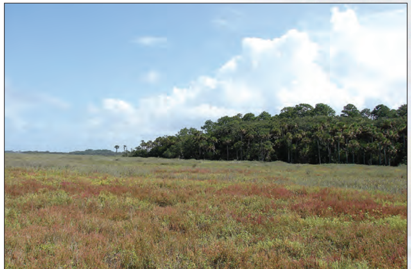
Top: A backfilled section of the perimeter ditch after excavation. Bottom: Salt marsh with saltwort, glasswort, and brushy seaside oxeye after restoration.
