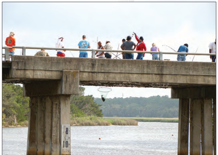
Top: The Tomoka River bridge, 1956, from the south approach of U.S. 1. Photo from Florida Memory website in the Florida Archives. Bottom: The Tomoka River bridge on the Old Dixie Highway, April 16, 2009. Photo by C. DuToit.
