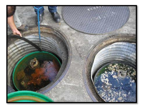
Maintenance - Water in excess of one inch in sumps or spill buckets or any regulated substances must be removed within 72 hours of discovery.
