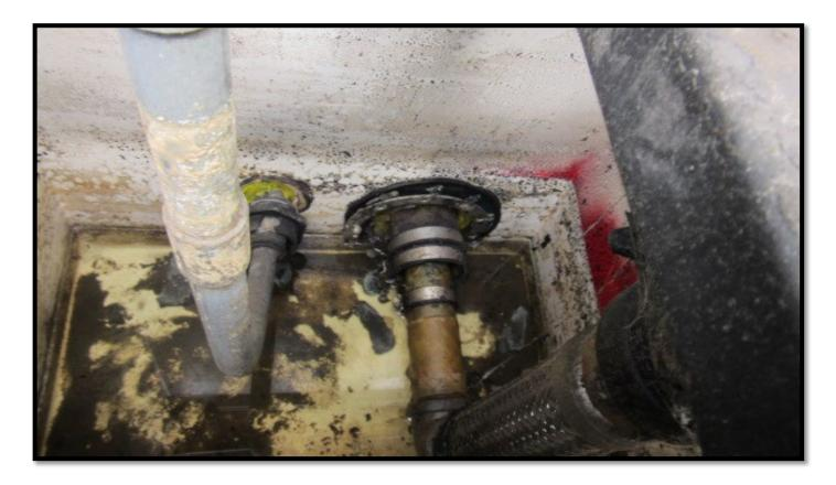
Piping and dispenser sumps that use electronic release detection must also be visually inspected every six months.
