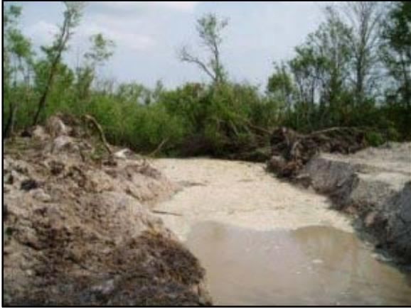
Drainage ditch used to dewater clay-filled areas
