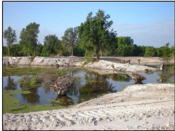
Earthmoving completed in East Waterfowl Area, with inverted tree stumps for bird roosts
