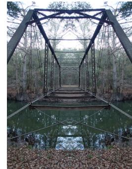
Bellamy Bridge, Photos Liz Sparks
