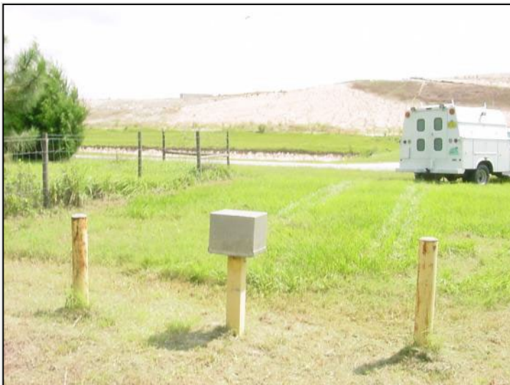
Figure 37. Which well is the correct one? It is important to ask the well owner if there are multiple wells clustered together.
