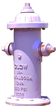
This purple fire hydrant is supplied by reclaimed water from the City of Tallahassee's Tram Road Reuse Facility.
