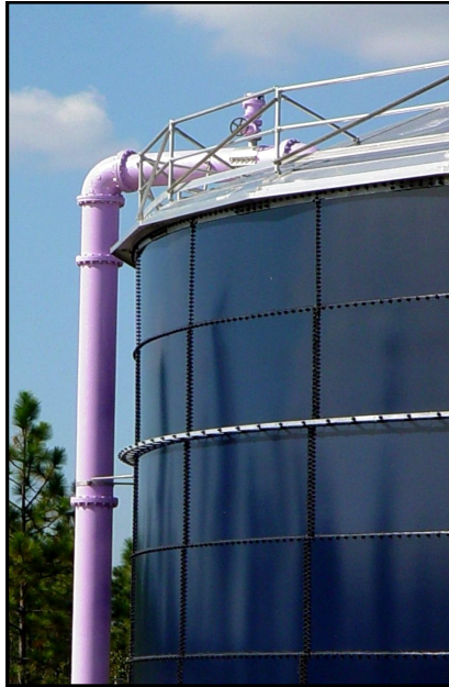
Reuse Storage Tank at Spencer WWTF (Photo by Shanin Speas-Frost)
