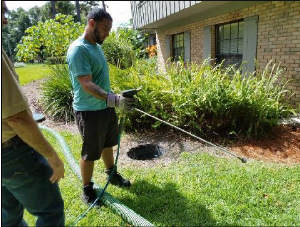
Re-Distribute the Sulfur Media Using a Pressure Washer 8/1/2019
