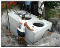
settling. After detention multiple chambers in overflows water the baffle box into the stormwater pipe. Most baffle boxes are buried in-line with the storm drain system, leaving only manhole covers visible from the ground
