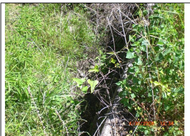
Trib. 5 just West of SR 65 on SR 65A - Dry
